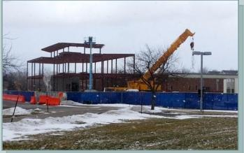
The steel for the B-21 expansion continues to rise out of the ground. About <sup>3</sup>/<sub>4</sub> of the steel is now up. The final one story portion of the structure will be erected in the next two weeks. The air handlers and electrical transformers were put into the basement concurrently with the steel erection so we will be ready for the warm summer days, even if we don't have any exterior walls at that point..... The construction of the
