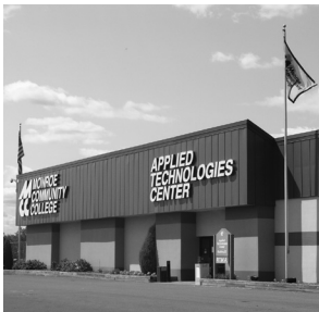
Applied Technologies Center 2485 W. Henrietta Rd. Rochester, NY 14623 585.292.3725
