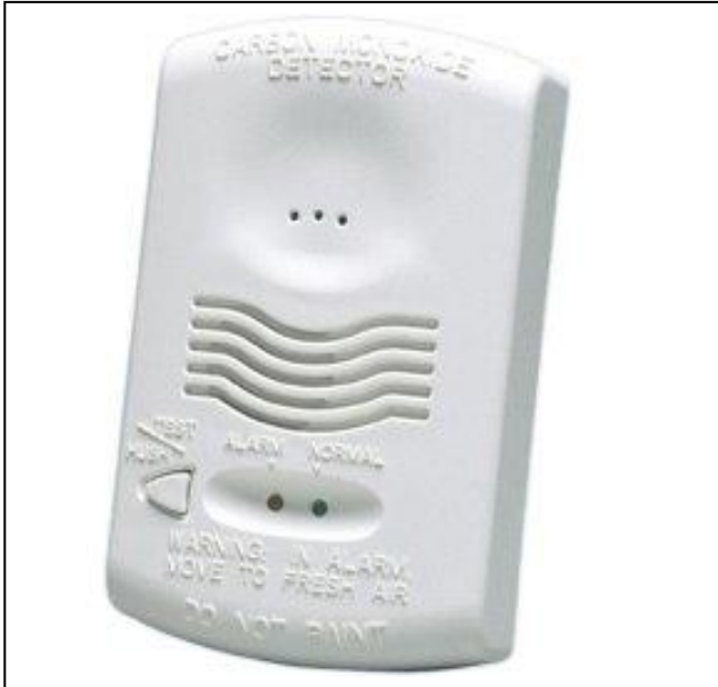
This photo shows the Carbon Monoxide detectors installed.
