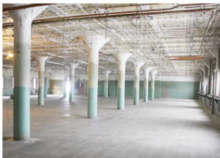
Walls, ductwork, ceiling, and carpet have been removed and asbestos abatement has been completed on the sixth floor to prepare for main construction.
