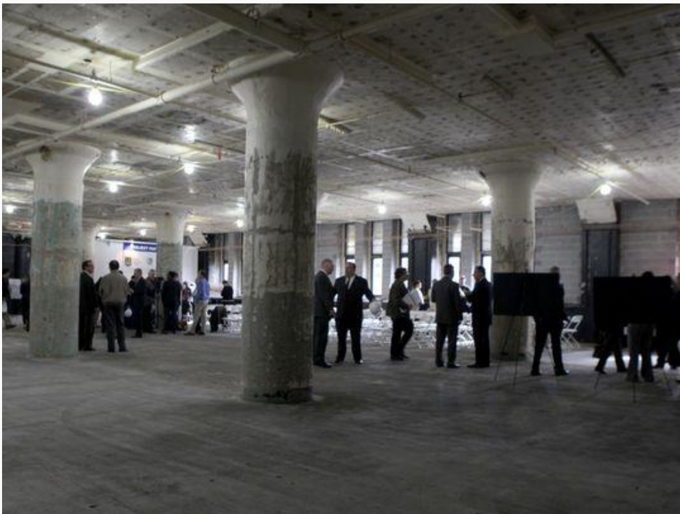
County Executive Maggie Brooks and MCC President Anne M. Kress held a press conference Oct. 20 to commence construction on Monroe Community College's new downtown campus. (Photo: MAX SCHULTE/@maxrocphoto/, STAFF PHOTOGRAPHER)
