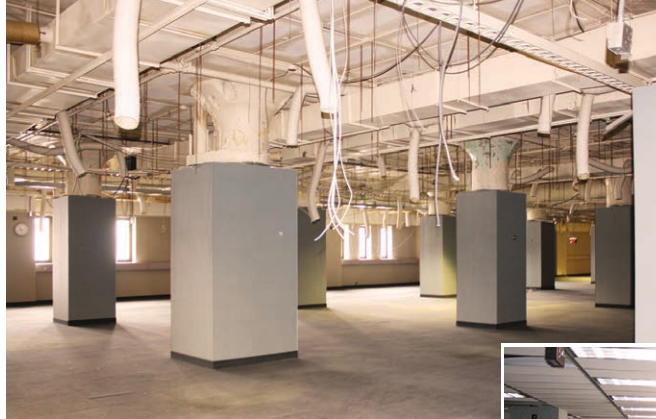
Ceilings, carpet, furniture, light fixtures, exit signs and some utility conduits (left) have been removed to prepare the area for asbestos abatement.
