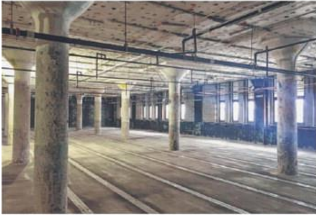
Fifth floor of site.
